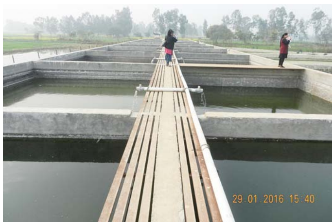
A view of Pangasius grow-out cemented tanks re-circulatory system with centrally placed iron frame and water supply at Nilgri village, Jahangirabad, Barabanki district, U.P.
